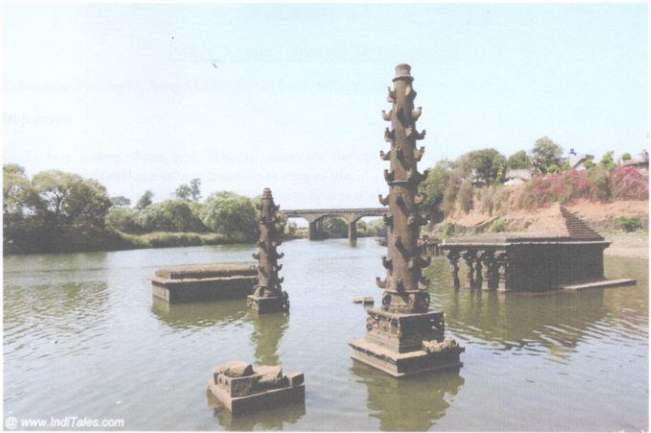
Panchganga River, Kolhapur
