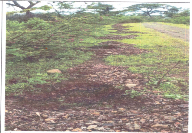
Pits dugged parallel to walking track for plantation near Kalamba lake site.
