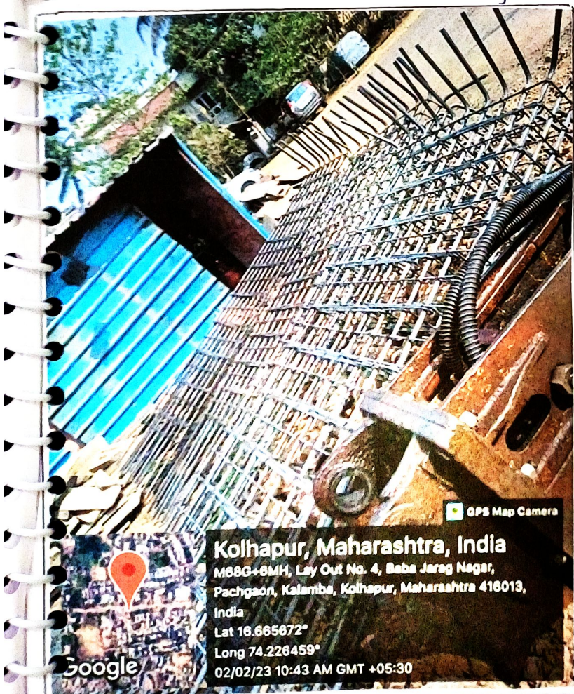
column c8, c9, c4 as I checked according to structural drawing
