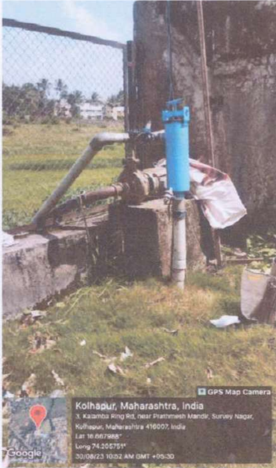
10 HP Motor- Water Lifting Pump Arrangements.
