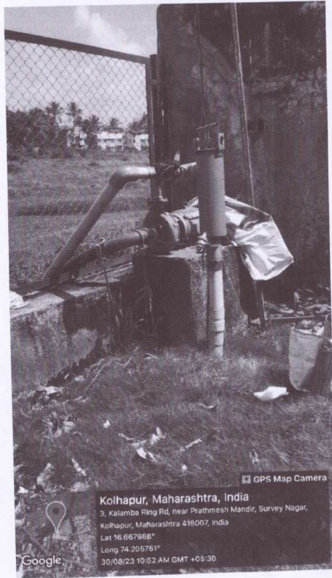
Fig: Waste Water Lifting Pump arrangements
