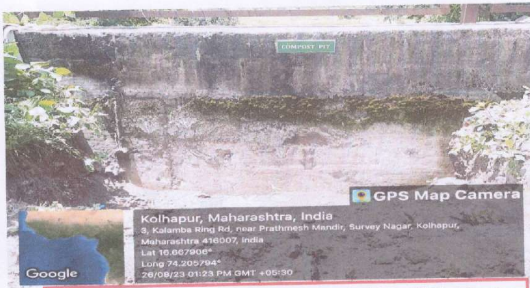
Compost Pit with Standard Dimensions (Depth=1.0 m , Width=2.0 m & Length=2.0 m)
